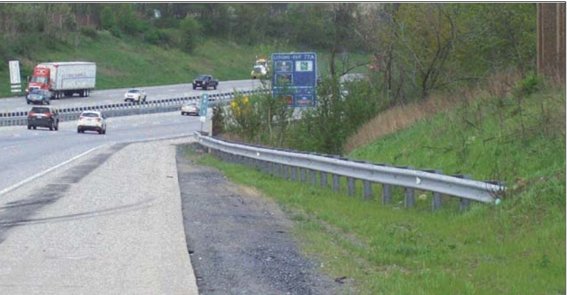
TYPICAL BURIED-IN-BACKSLOPE TERMINAL SINGLE RAIL
