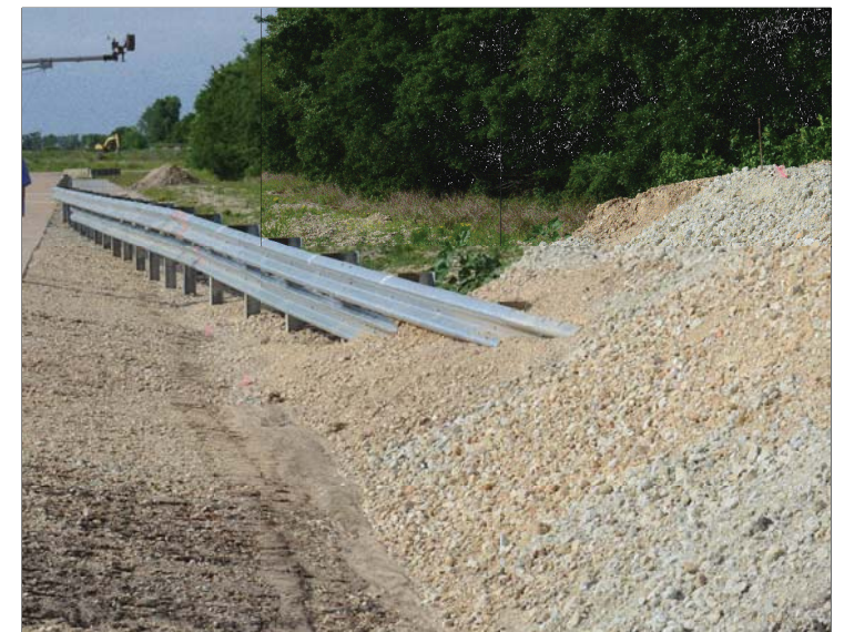
TYPICAL BURIED-IN-BACKSLOPE TERMINAL DOUBLE RAIL
