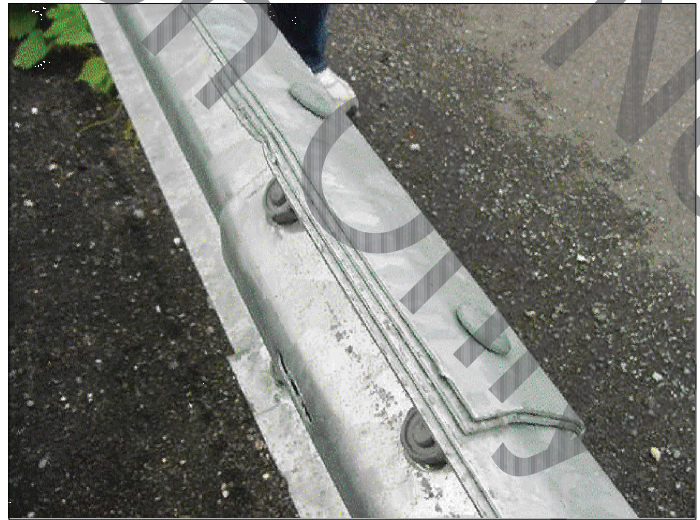
TYPICAL NESTED PANEL MID-SPAN SPLICE
