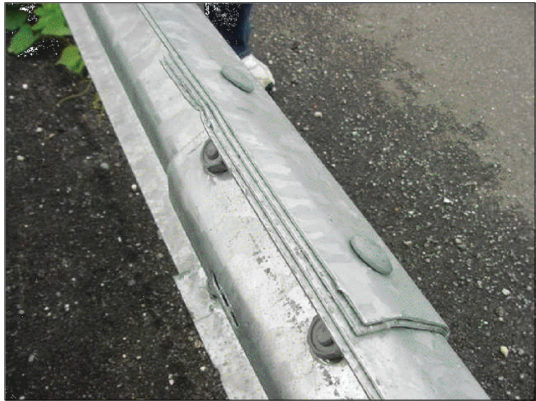
TYPICAL NESTED PANEL MID-SPAN SPLICE (SEE NOTES 2, 3, AND 4)
